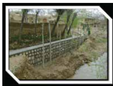
A Retaining wall in Donkqala village
