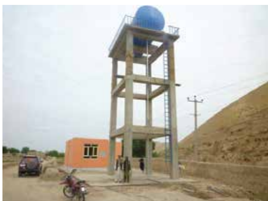
Water Supply Network, Shirintagab, Faryab province.
