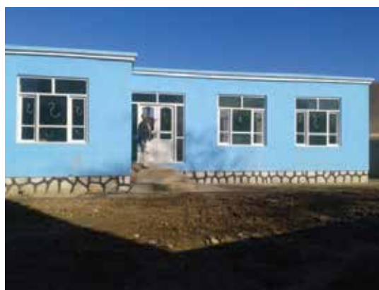
School building Construction, Shirintagab, Faryab province.
