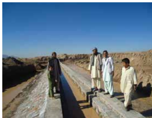
Canal Construction, Samalan Ulia, Shindand, Herat province.
